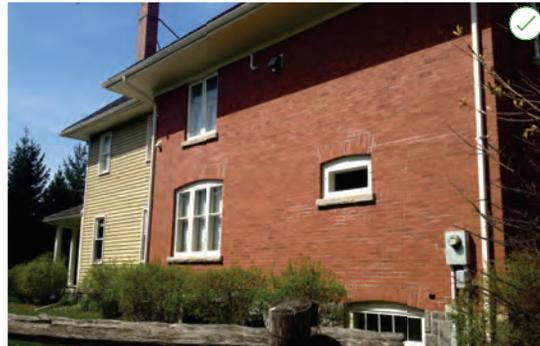
DO: addition is set back, windows in proportion, and cladding material compliments the original brick.
