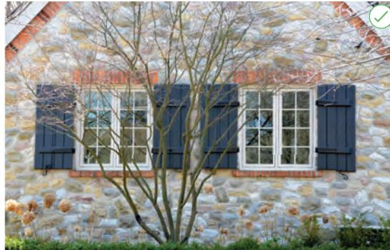
DO: this photo shows operable storm shutters that are appropriately sized for the window.
